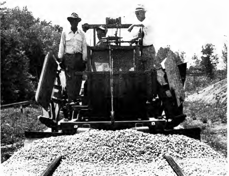
Machine for regulating and plowing ballast.
